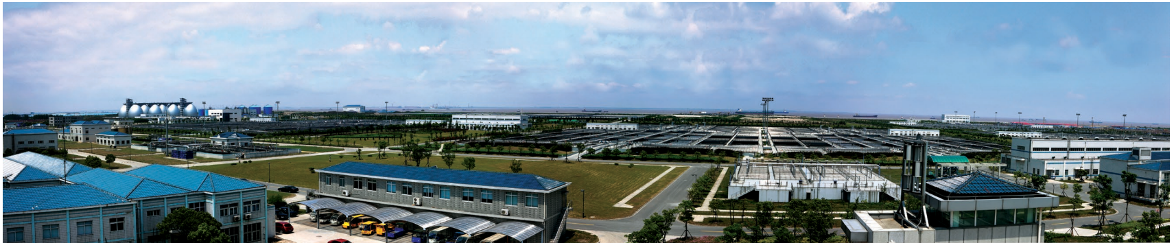
The largest waste water treatment plants in Asia The Shanghai Bailonggang Wastewater Treatment Plant
